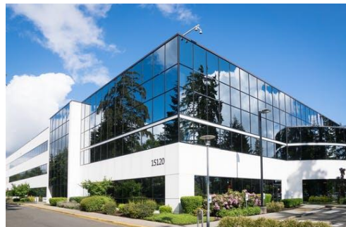
Facilities Maintenance (commercial)
