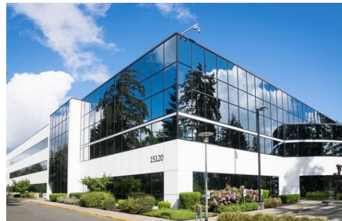
Facilities Maintenance (commercial)
